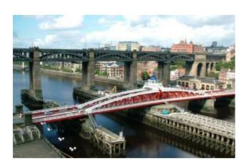
Newcastle's famous bridges across the Tyne are probably known to us all, but William Armstrong's 1876 hydraulic swing bridge has struck a problem. It has not opened for 18 months and an attempt made on 15<sup>th</sup>. August ended in failure as the mechanism failed to operate.
