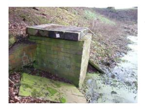
This shaft lies immediately beside the water and has a heavy wooden cover. Inside it is almost full of water – up to the level of the moat. It is likely that this was on outlet from the moat but no details can be seen. It might be part of the Water Feature (item 3a) or give access to a drain valve.
