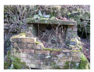
Item 6a. This decayed brick chamber is a collection chamber for sewage. At least two drains enter from the castle and the outlet is a cast iron main leading to item 5. One difficult to explain curiosity is the location of a gate valve in the cast iron main a few feet from the collection chamber. Normally sewage pipes dare not valved.
