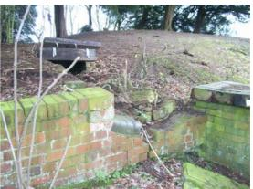
Item 3a is a circular blue brick shaft with a shaped lip facing the moat. The bricks have curved faces. Abutting the lip is a brick lined channel leading
