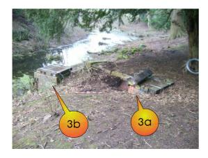
Close by the location of the lost footbridge are two brick shafts, a brick lined channel and some other brickwork. Both shafts have the heavy wooden covers which can be seen in the photographs.
