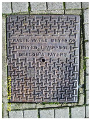
Now Mr. Deacon was a late 19<sup>th</sup> century civil engineer who is credited with bringing the first water from Wales to Liverpool. He also invented the first recording water meter – a clockwork device that recorded the changing water use over a 24 hour period.
