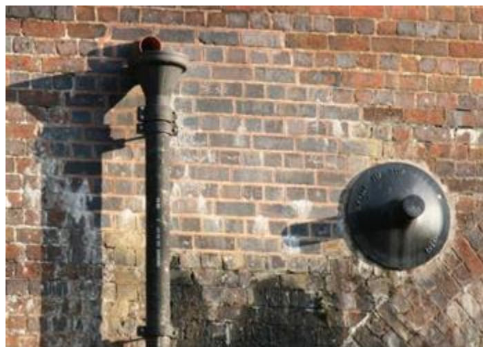
Modern tie plate with the date 2008 cast into it - Mill End, Kenilworth
