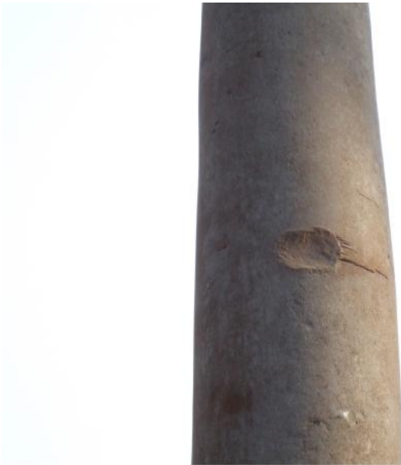
Pillar has been used for target practice by the Army in the past
