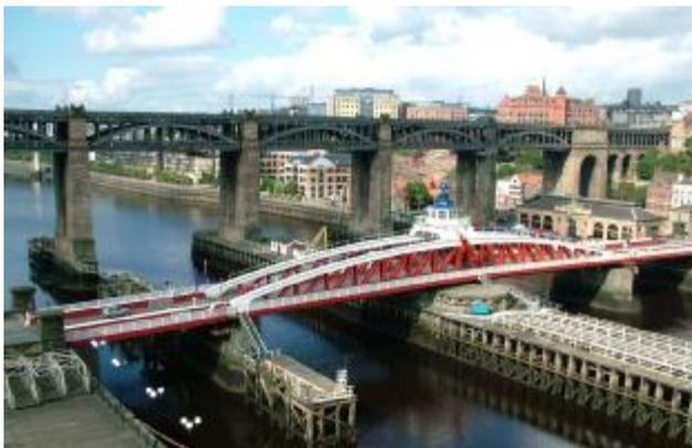
Newcastle's famous bridges across the Tyne are probably known to us all, but William Armstrong's 1876 hydraulic swing bridge has struck a problem. It has not opened for 18 months and an attempt made on 15<sup>th</sup>. August ended in failure as the mechanism failed to operate.
